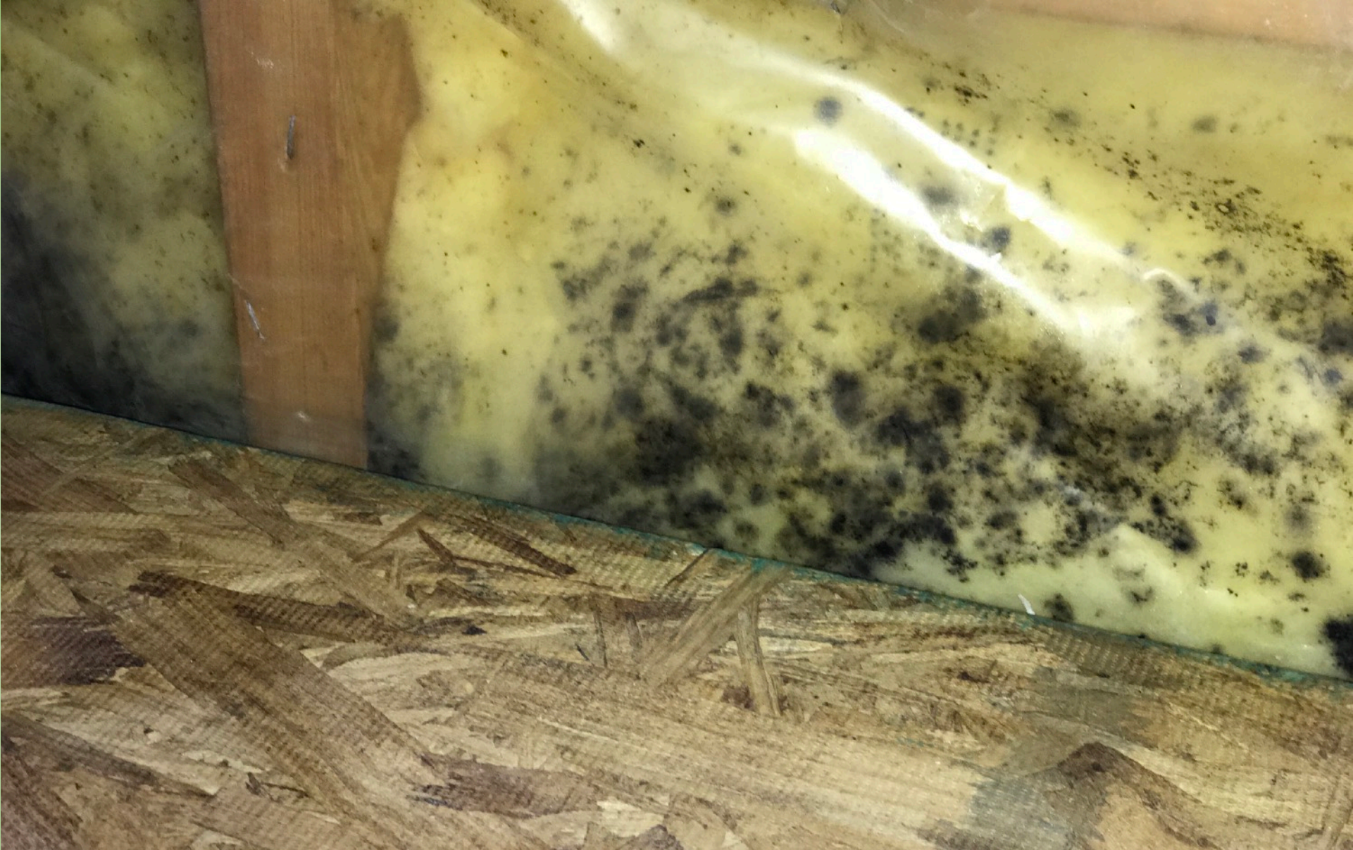
Poly-barrier used in warm climates cause mold behind walls
