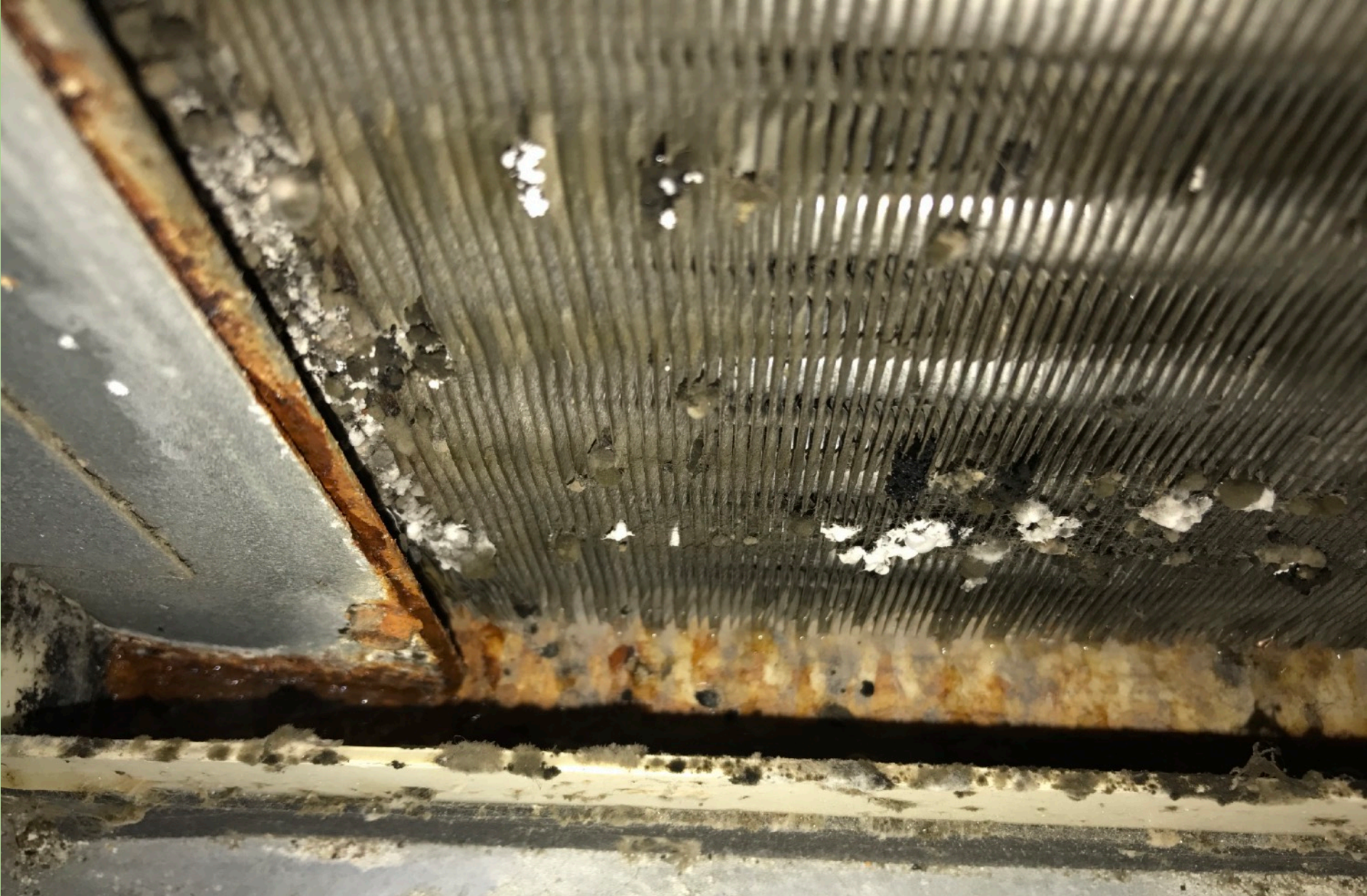
Mold on Coil Fins of AC
